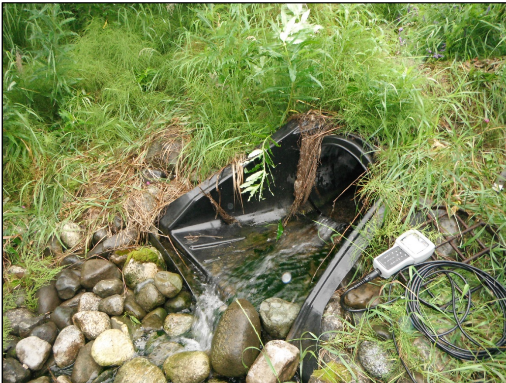
Photograph 2. Outfall SWM02 (847-1), Home Depot on Abbott Road.
