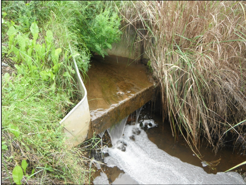
Photograph 5. Outfall SWM05 (207-1), East 56 th Avenue at Save School.
