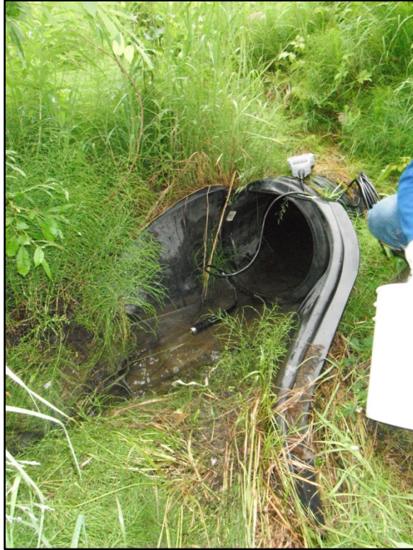
Photograph 1. Outfall SWM01 (1040-3), Ridgemont Drive.
