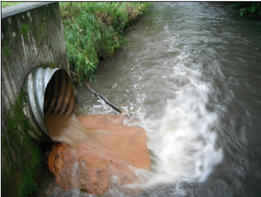
Photograph 10. Outfall SWM10 (525-2), Eagle Street at Chester Creek.
